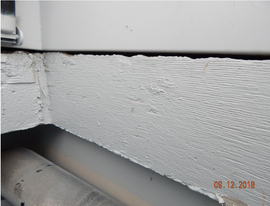
Reinforced Concrete Roof Deck
