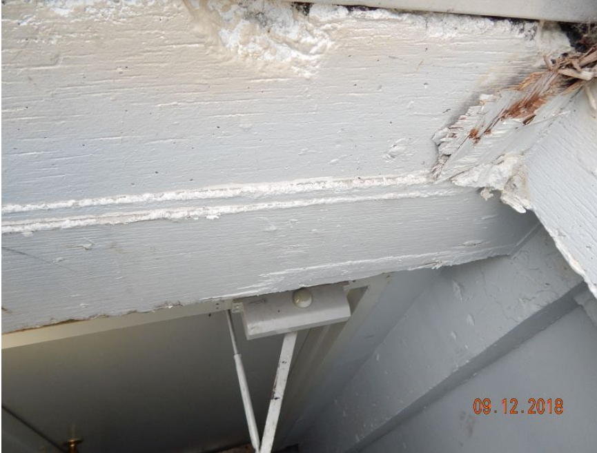
Reinforced Concrete Roof Deck
